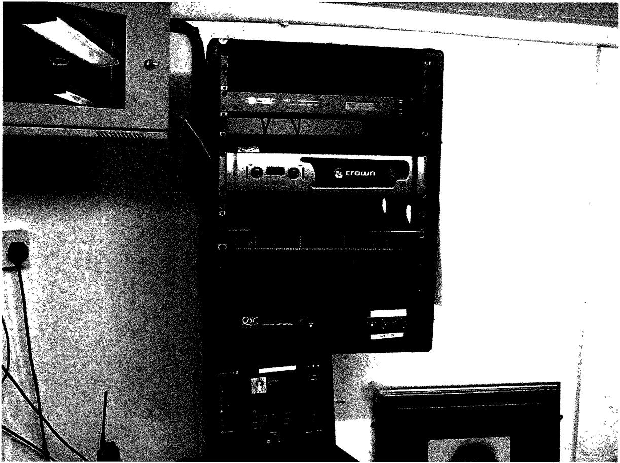
Figure 1: Equipment rack is located in basement office. Note: AVC2-D limiter at top of rack. Mixer/zoner and all gain controls behind tamperproof panels.
